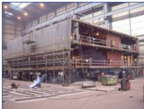
Accommodation unit being fabricated
