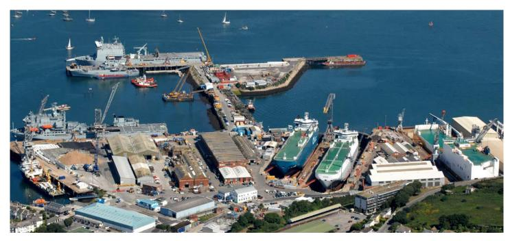
FALMOUTH, IN THE COUNTY OF CORNWALL, HAS A LARGE NATURAL DEEP-WATER HARBOUR AND ONE OF THE LARGEST COMMERCIAL SHIP REPAIR COMPLEXES IN THE UK. WE HAVE THREE LARGE GRAVING DOCKS AND EXTENSIVE ALONGSIDE DEEP WATER BERTHING PROVIDING CAPACITY FOR VESSELS OF UP TO 100,000 DWT.
