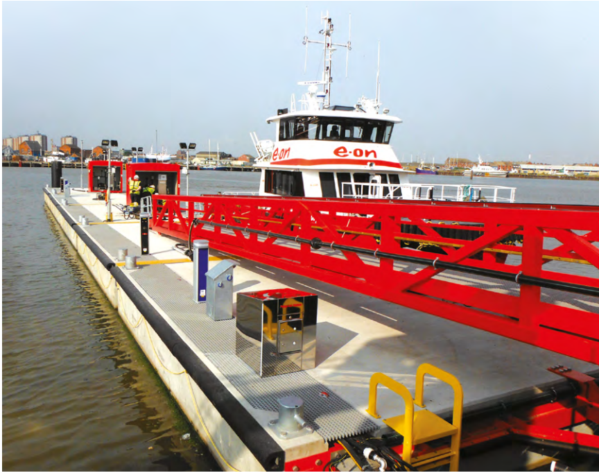
Grimsby, 2015, 6m wide fully serviced CTV pontoon with fuel, water, pump out, task lighting & top entry service ducts.
