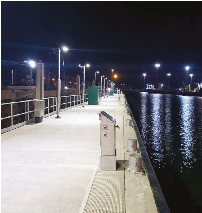
Barrow at night, task lighting.
